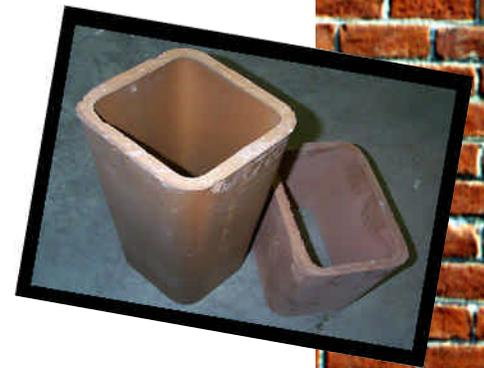
Clay flue tiles are required because building codes specify that the liner system must extend 2 inches above the top of the chimney.
