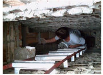
All openings and or weak areas in the chimney structure are braced and reinforced before the former is installed.
