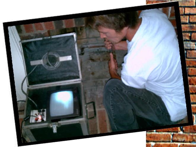
**Step 1:** We inspect the chimney both visually and with a video inspection camera and record our findings on a condition report.
