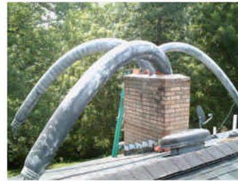
The Supaformer is then inflated and centered within the flue with the use of spacers. The chimney in this picture will have three new flues.
