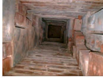
The existing clay flue tiles are removed from the chimney to make room for the new system.
