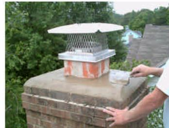
A new crown is poured at the top of the chimney to seal out water.
