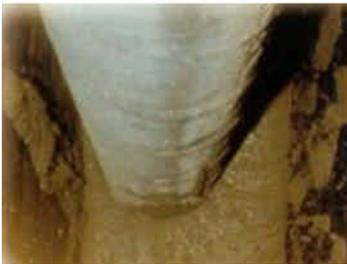
The Supaflu mix is prepared on site and is then pumped into the chimney from the top. The mix is pumped between the Supaformer and inside of the chimney wall.
