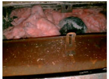
In addition to the fireplace opening being sealed off, the area around the damper plate is also sealed off to prevent mix from falling into the firebox.
