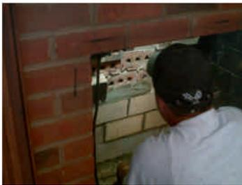
Depending on the condition of the back wall one or all three walls will be rebuilt.
